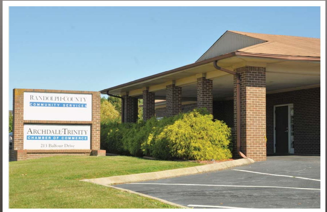
Randolph County Community Services Building
